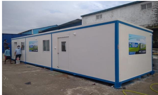
Fig 1. FRP composite quarantine unit made in India (NMB TATA Steel ltd.)
